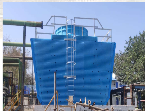
HANDRAIL AND LADDER
